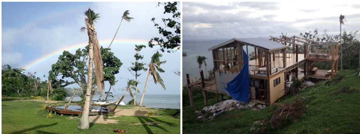
Damaged infrastructure on Koro Island. ©Akanisi Caginitoba/WCS
